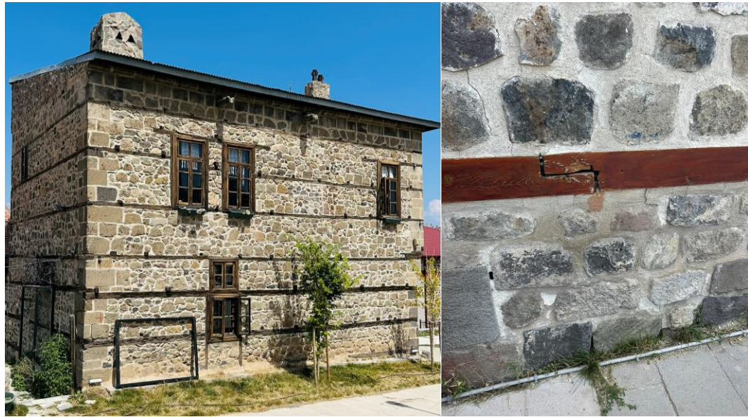
(a) Use of tie beams in a stone masonry structure
